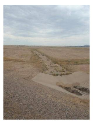
**Photo 3.** View of northwest end of airport runway area showing drainage feature to direct surface runoff to Powerline Floodway; photo taken facing southeast.
