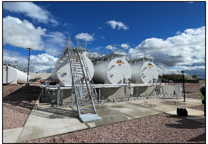
Three New 50,000 Gallon Aviation Fuel Storage Tanks Expands On-Airport Storage Capacity to 400,000 Gallons
