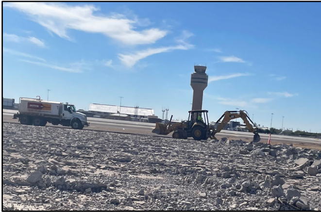
Demolished Concrete Being Removed from the Runway
