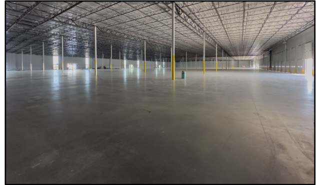
SkyBridge Arizona 250,000 Sq. Ft. Building Interior
