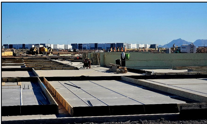
Wall Fabrication for Gateway Commerce Center III
