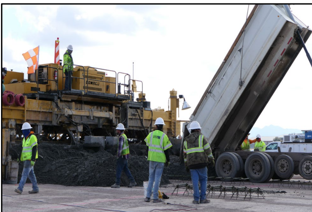
Concrete Being Placed on Runway 12R/30L
