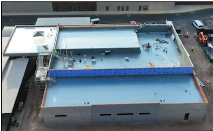
New TSA EDS Facility Under Construction
