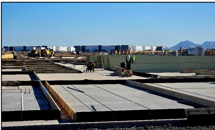
Wall Fabrication for Gateway Commerce Center III
