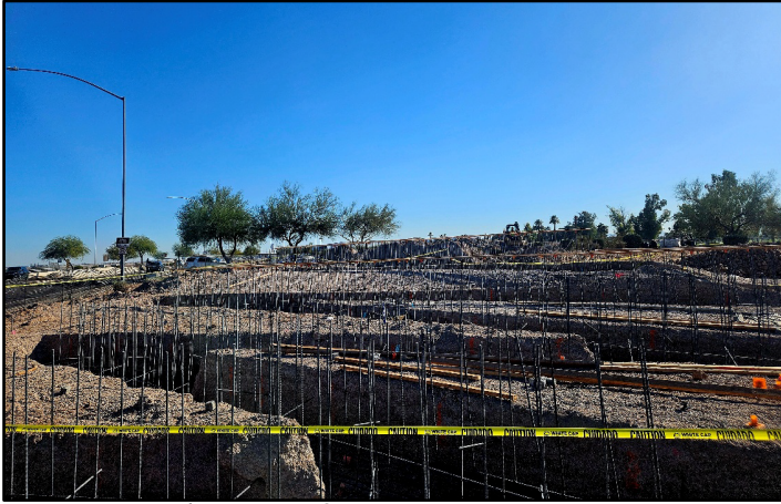
Footings and Framing for New Entrance Sign
